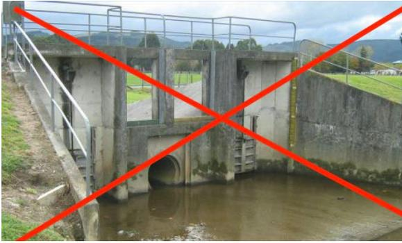
After the 1976 flood a detention dam was built to hold water from Heretaunga back so that during a big storm the water level in Hulls Creek would be low, allowing the Pinehaven Stream to empty out into Hulls Creek, reducing flooding in Silverstream. Council's model assumes a high water level in Hulls Creek (as if the detention dam isn't there), increasing flooding in Silverstream.
