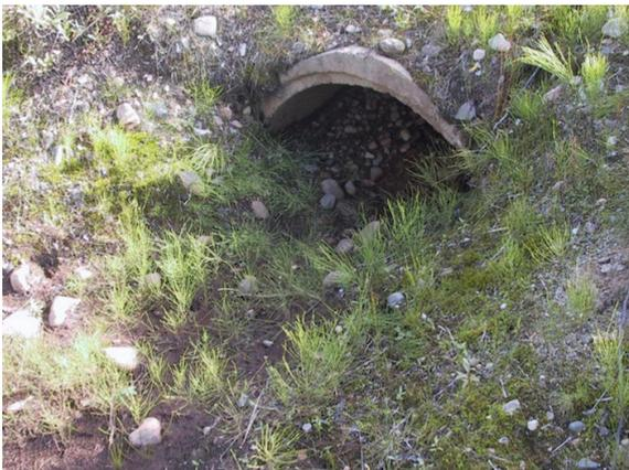
Council's flood model assumes all culverts up to 1.2m diameter are 100% blocked, sending floodwater out over roads and properties. This is one way of allowing for blockages in a storm.
